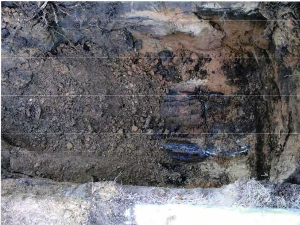
Picture 2: UST 879Cobia excavation in progress.
